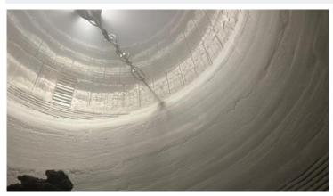
RHI Magnesita Seven Refractories, the joint venture between RHI Magnesita India and Seven Refractories, has successfully executed the job of monolithics application with robotic shotcrete technology to help resume the operations of Blast Furnace at one of the large steel plants in Eastern India.
